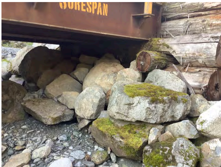
Left Bank Abutment when facing downstream
