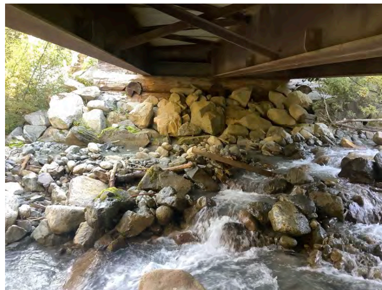
Right Bank Abutment when facing downstream
